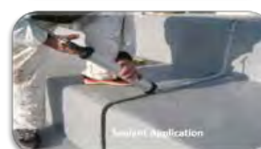
STP Tank Waterproofing
