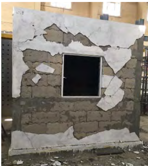
Damage Pattern from Lateral Load Test
