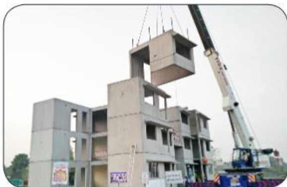
4. Prefabricated Sandwich Panel System
