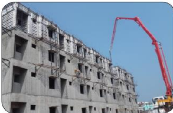
5. Monolithic Concrete Construction
