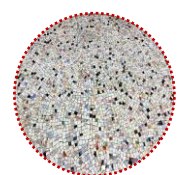
China Mosaic Tiles on Roof
