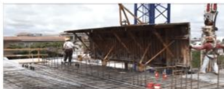
Kicker form of tunnel formwork panel
