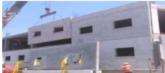
Precast concrete wall (Panels)
