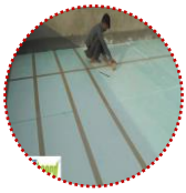
EPS Insulation on Roof
