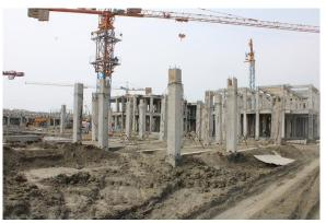
**Precast Column Erection**
