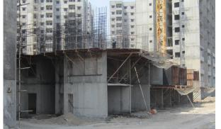
Tunnel formwork panel slab and wall casting
