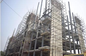
Assembly of LGS Frames and Construction of Wall
