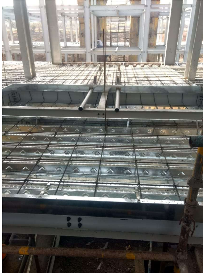
Services & Reinforcement Laying
