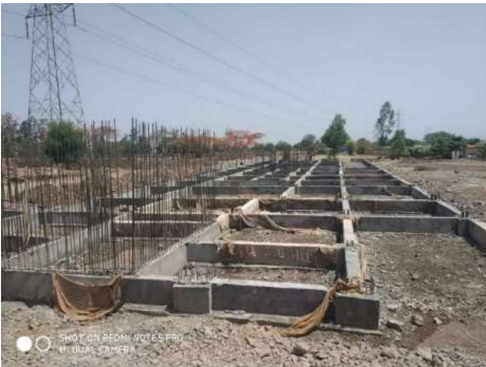
RCC COLUMN UP TO PLINTH LEVEL
