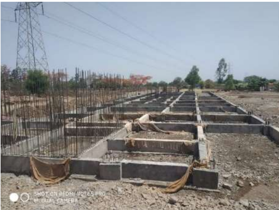
RCC COLUMN UP TO PLINTH LEVEL
