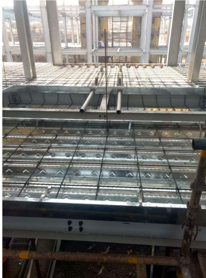
Services & Reinforcement Laying
