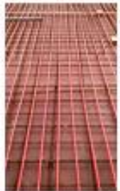
RADIANT COOLING Radiant cooling handles the sensible heat load
