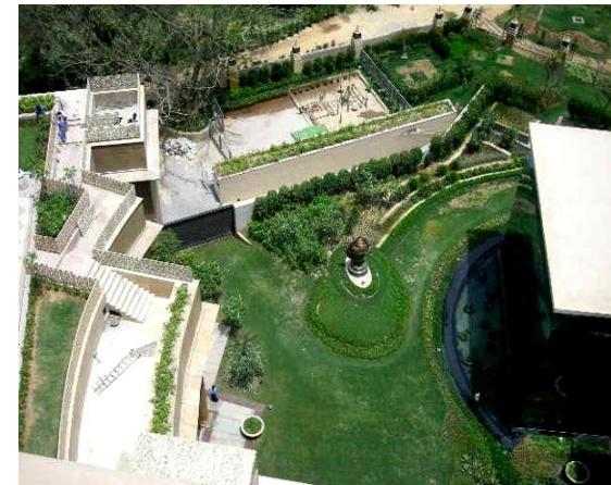
Combination of high SRI coating & roof garden in Hotel Leela Palace, Delhi
