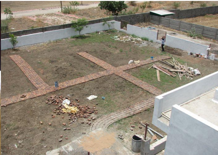
Broken bricks being used for paving Tatva, Indore - IGBC Platinum
