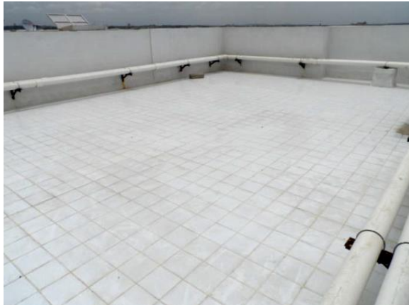
High SRI Tiles on Roof Raheja Vistas, Hyderabad
