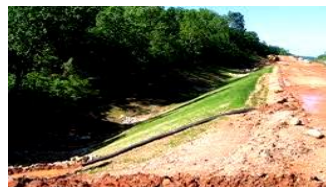
Topsoil covered with temporary Seeding
