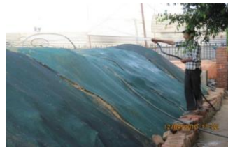
Topsoil covered with temporary Covering
