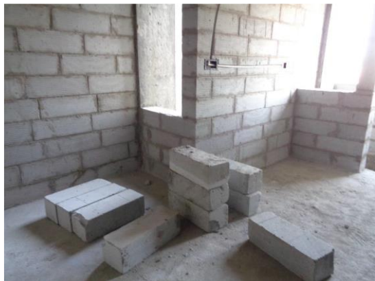
200 mm AAC block with U value – 0.7 \text{ W/m}^2\text{k}
