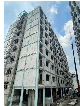
Steel Structure Prefabricated EPS Panel
