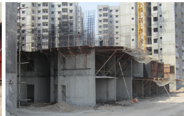
Building Using Tunnel Formwork
