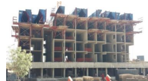
Building Using Tunnel Formwork
