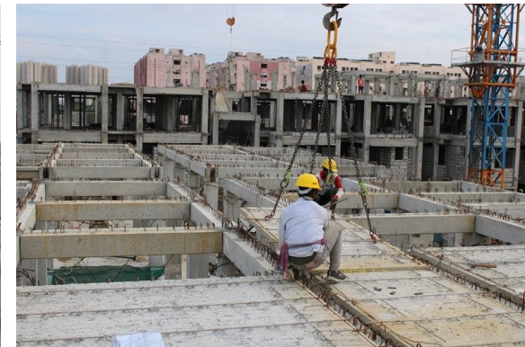
Precast Slab work
