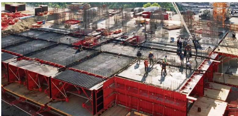
Tunnel formwork panel slab and wall casting
