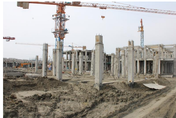
Precast Column Erection
