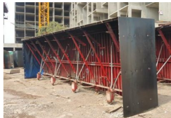
Tunnel formwork panel slab and wall casting
