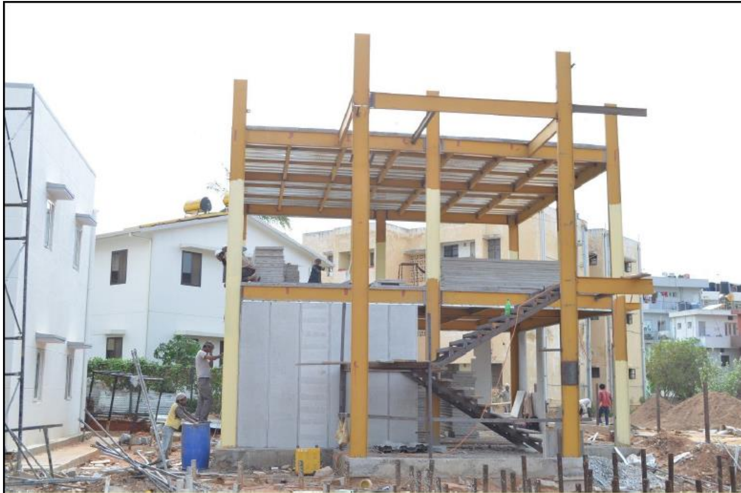
Steel skeleton with Aerocon panel infills
