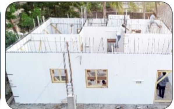
6. Stay In Place Formwork System
