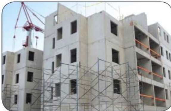
4. Prefabricated Sandwich Panel System
