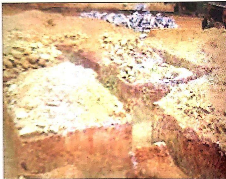
Good Soil (Hard strata recorded in shallow depth)
