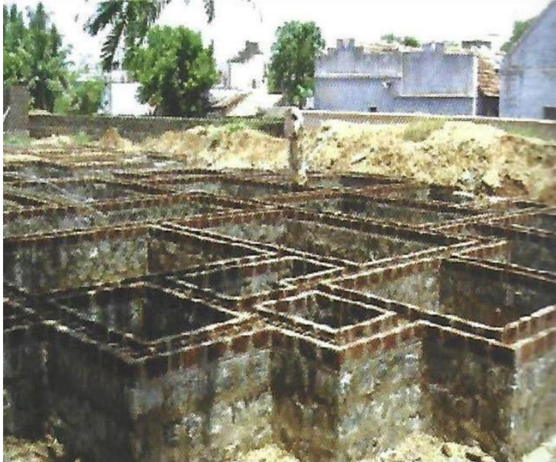
Example of proper RR masonry
