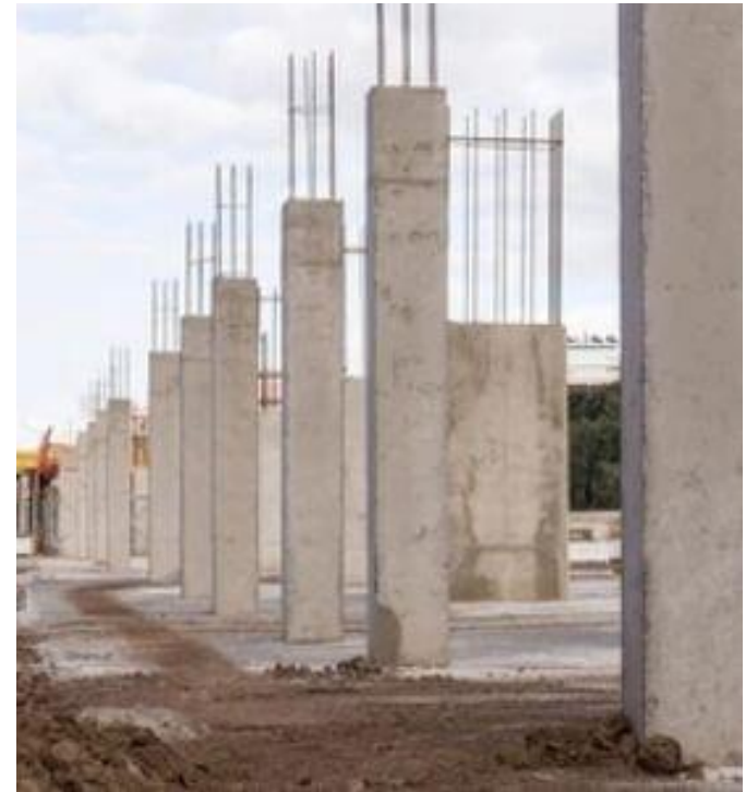
Example for proper column concrete
