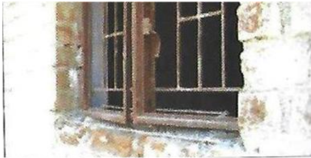
Improper marking of windows sill slab
