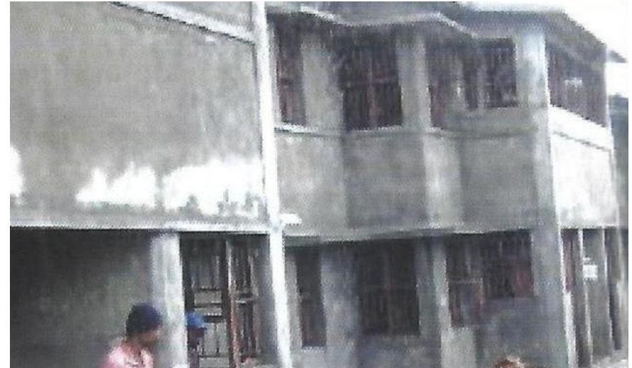
Example for proper plastering in hilly areas
