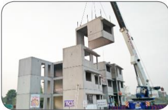
4. Prefabricated Sandwich Panel System
