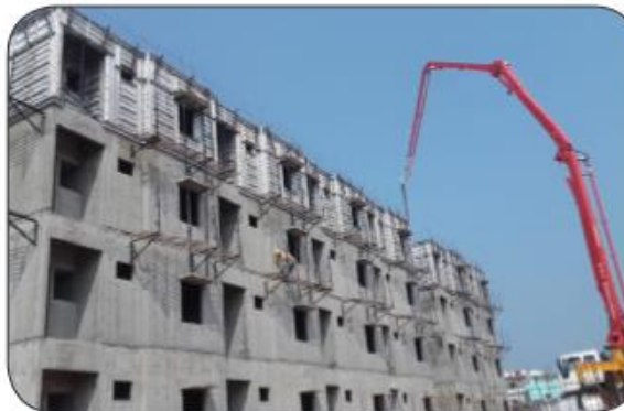
5. Monolithic Concrete Construction
