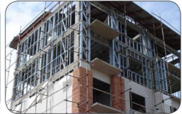
6. Stay In Place Formwork System
