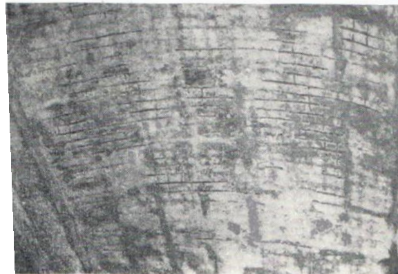
Corrosion damage to an Exposed ceiling of shell Roof
