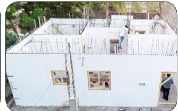
6. Stay In Place Formwork System
