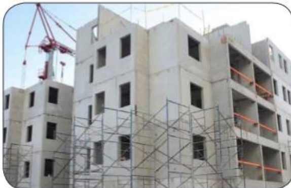
4. Prefabricated Sandwich Panel System
