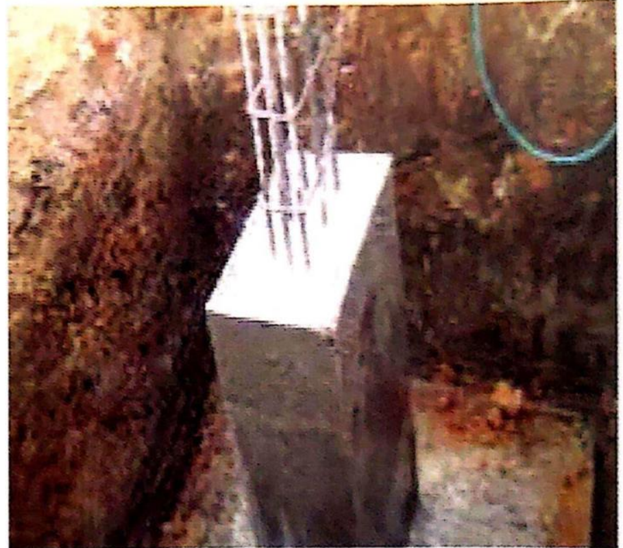
Column pedestal provided with proper cover
