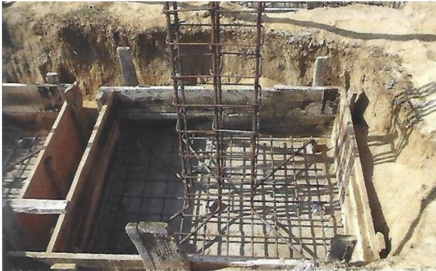
Method of positioning the foundation reinforcement
