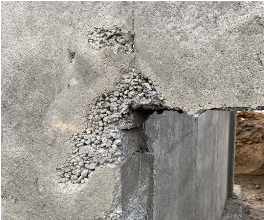
Poor quality of concrete due to improper water cement ratio
