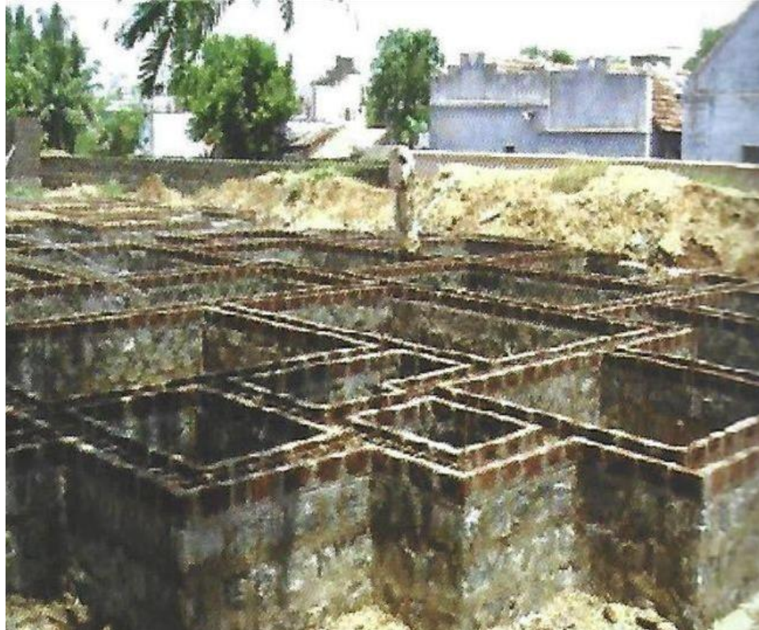
Example of proper RR masonry
