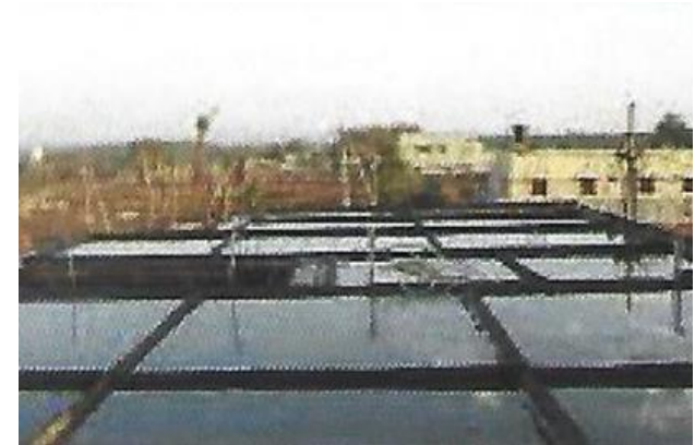
Pond curing for roof slab
