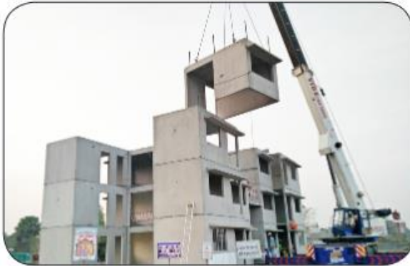
4. Prefabricated Sandwich Panel System
