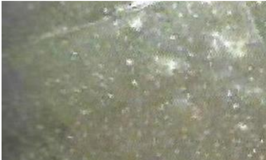
Proper hacking of roof slab before plastering
