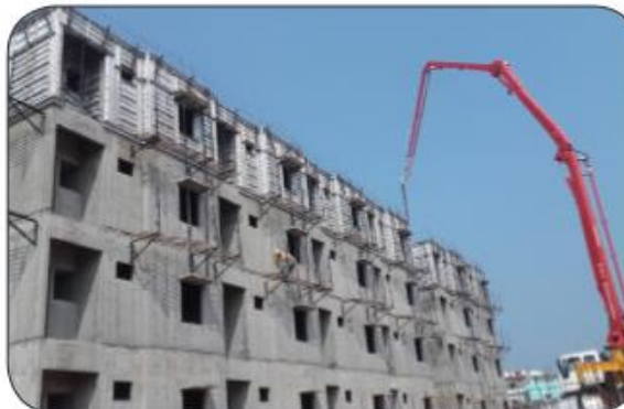
5. Monolithic Concrete Construction
