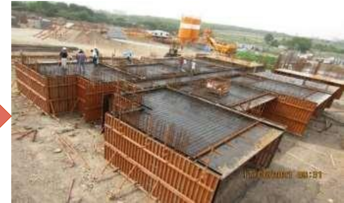
Assembly of Formwork
