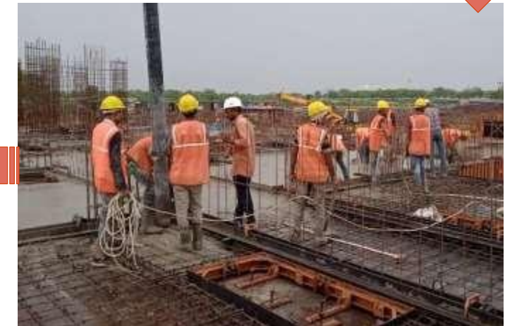
Concreting after Placing formwork
