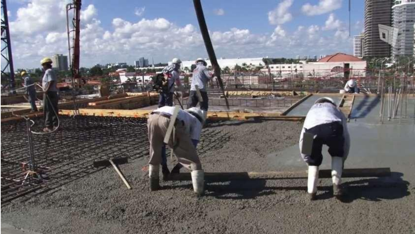
Placement and leveling of concrete
