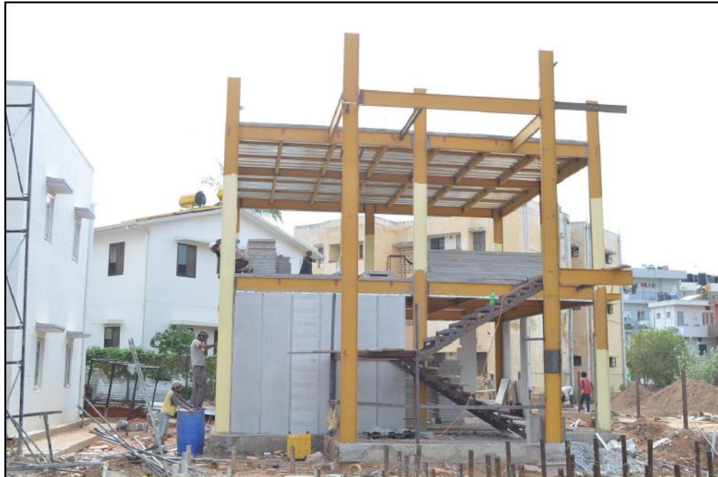
Steel skeleton with Aerocon panel infills
