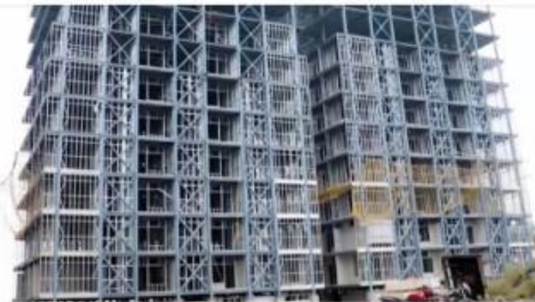
Assembly of LGS Frames and Construction of Wall
