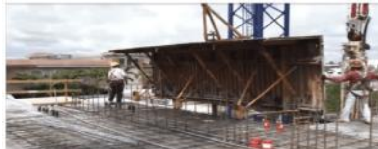
Kicker form of tunnel formwork panel
