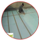
EPS Insulation on Roof
