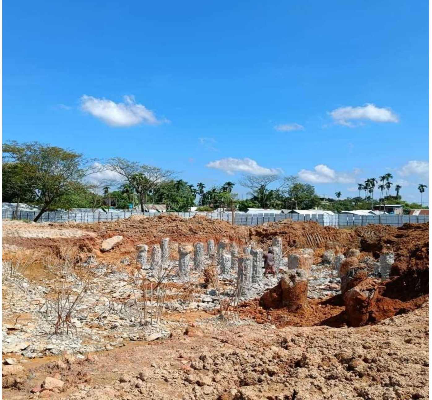
Excavation and pile head breaking
