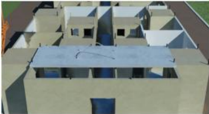
Construction and installation
