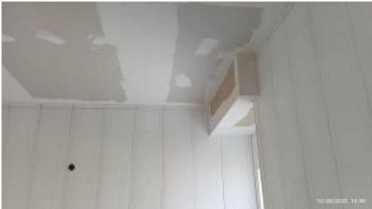
False Ceiling with Gypsum Board
