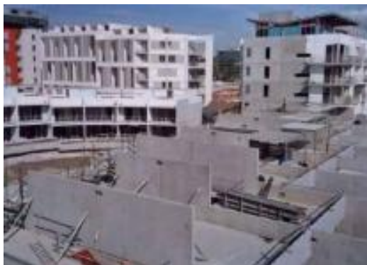
Installation of panels
