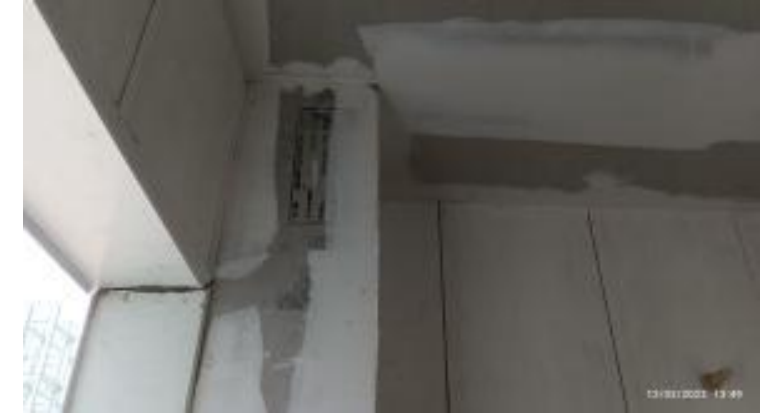
Structure Cover with Cement Fiber Board
