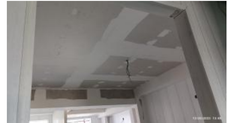
False Ceiling with Gypsum Board
