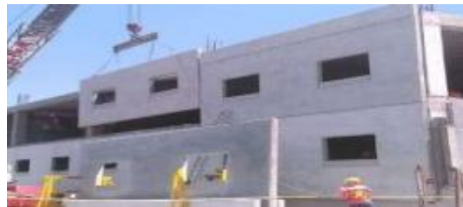
Precast concrete wall (Panels)
