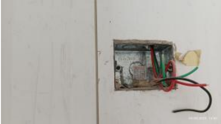
Electrical Switch Board
