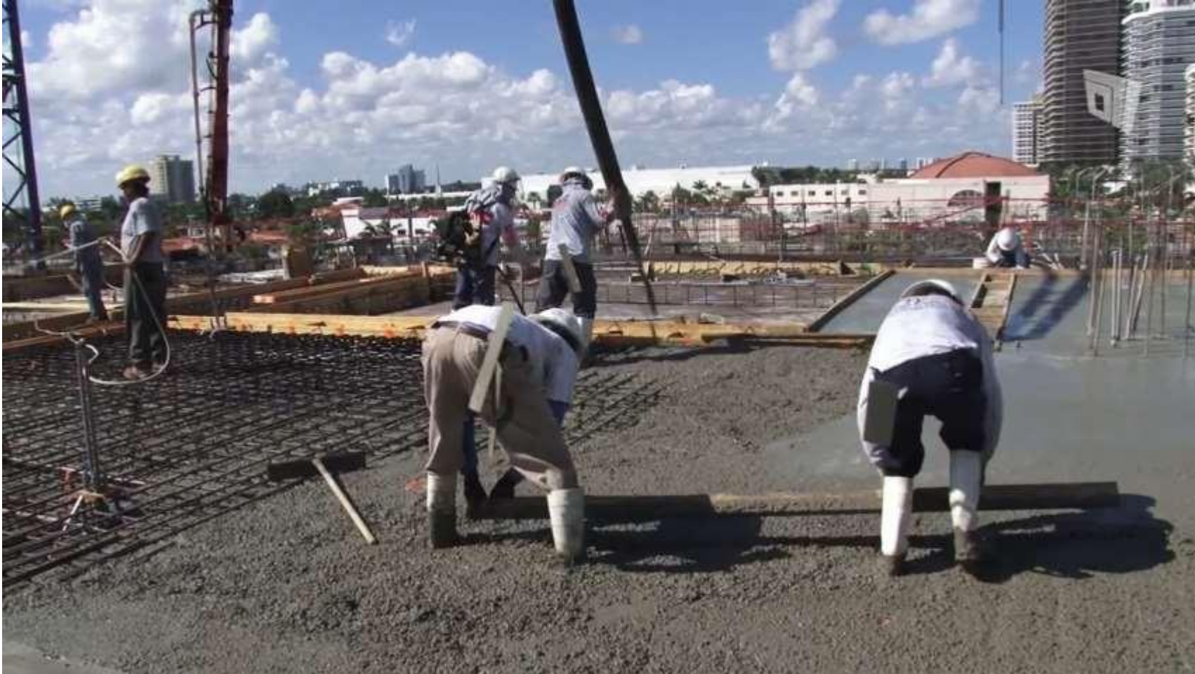
Placement and leveling of concrete
