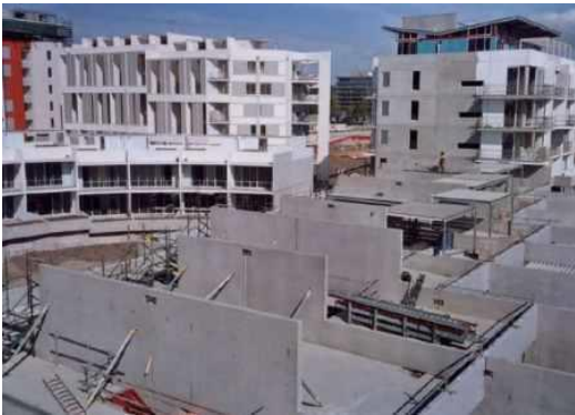
Installation of panels
