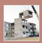
Precast Concrete Construction System – 3D Volumetric
