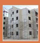
Prefabricated Sandwich Panel System
