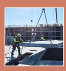
Precast Concrete Construction System – Precast Components Assembled at Site
