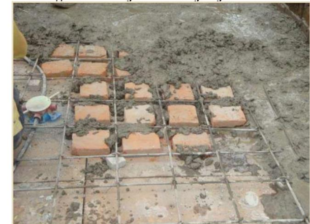
Figure 2 Reinforcement for filler slab
