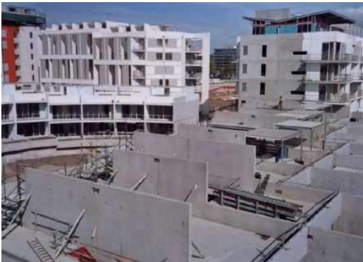
Installation of panels
