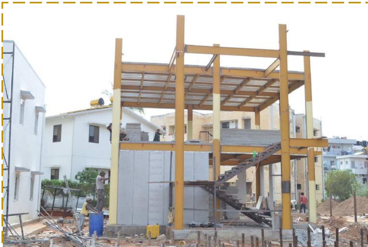
Steel skeleton with Aerocon panel infills
