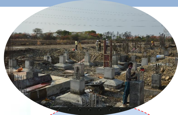
1. Substructure RCC Isolated column footing
