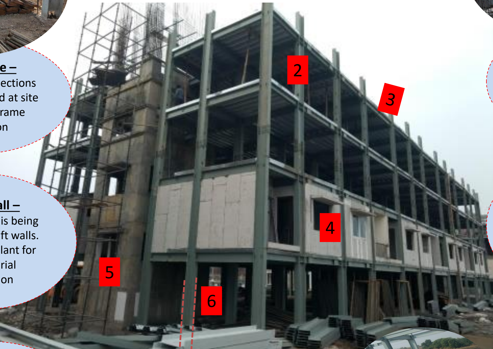
4. Walling System Factory made Prefabricated sandwich panels are being used for wall preparation
