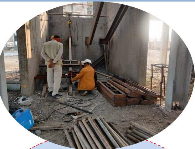
6. Staircase – Fabricated MS sections are being welded at site for staircase frame preparation
