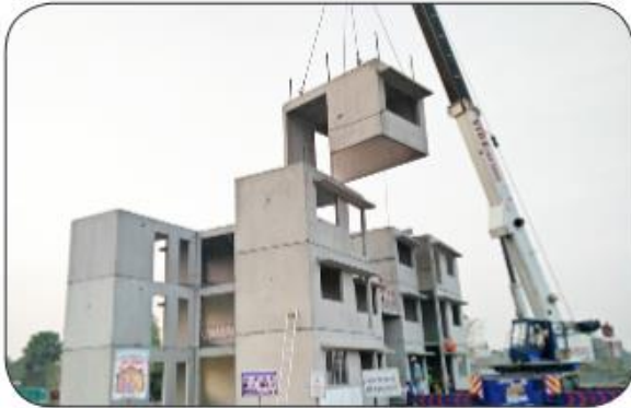
4. Prefabricated Sandwich Panel System
