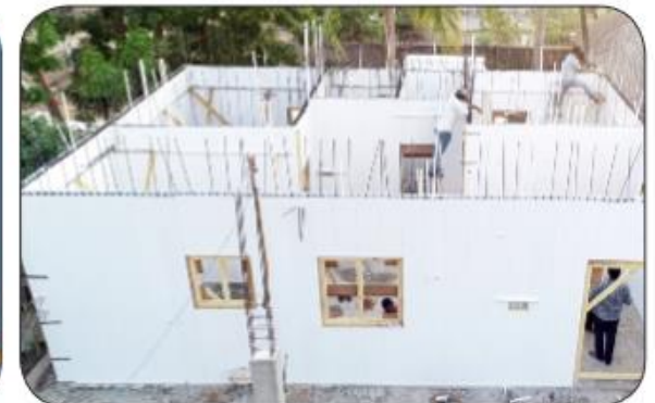
6. Stay In Place Formwork System
