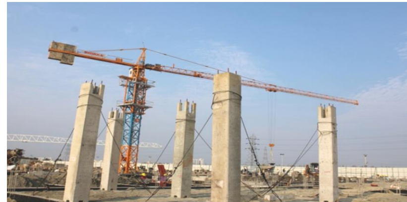
Ground Floor Column Work in Progress - March 2021
