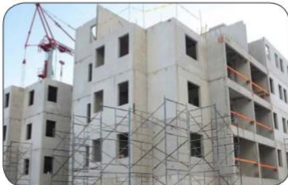
4. Prefabricated Sandwich Panel System
