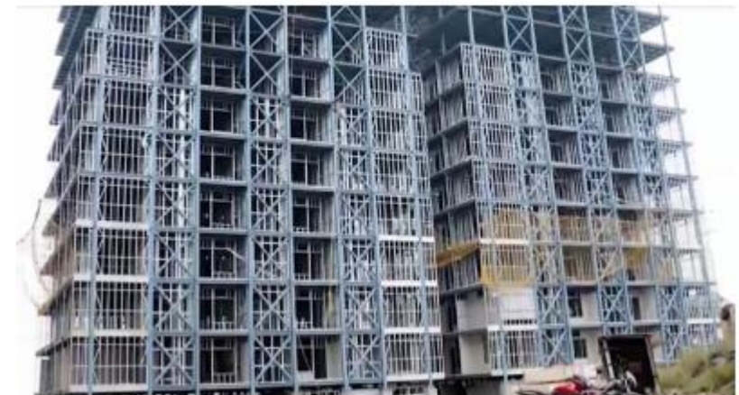
Assembly of LGS Frames and Construction of Wall
