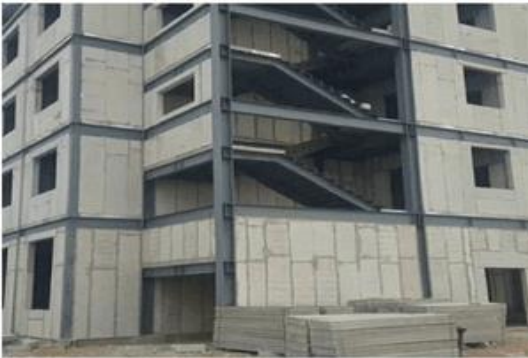
Steel Structure Prefabricated EPS Panel
