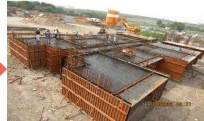
Assembly of Formwork
