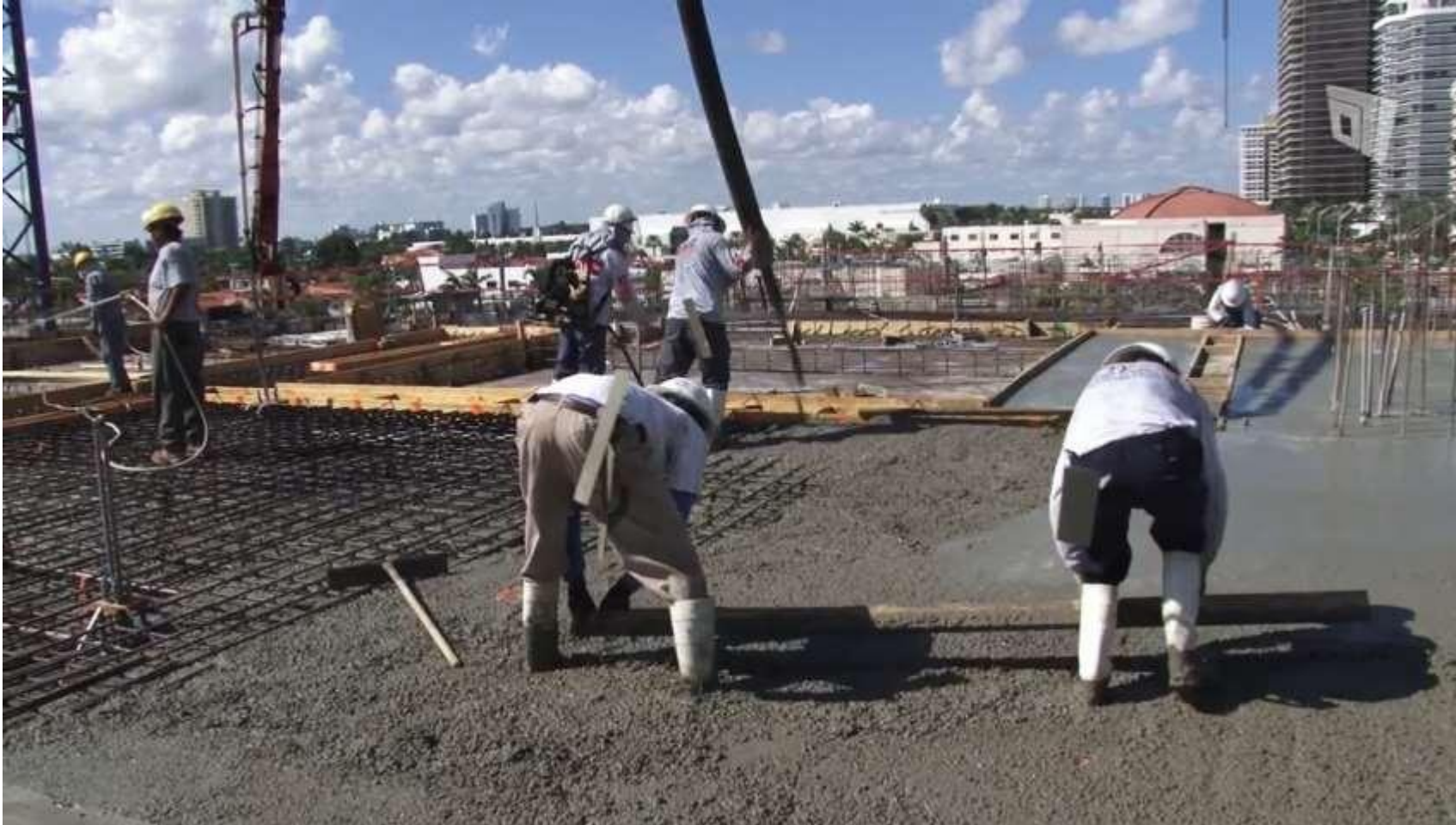
Placement and leveling of concrete
