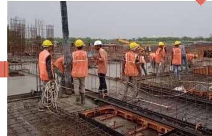
Concreting after Placing formwork
