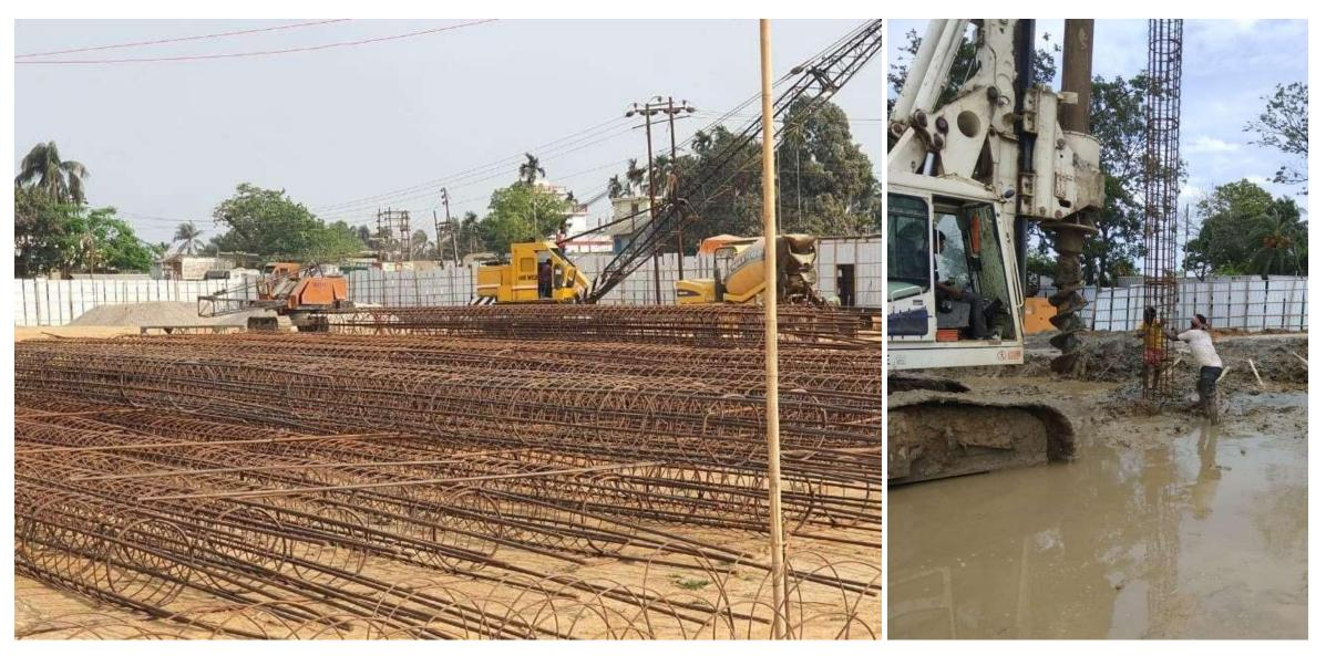
• Steel Cages with helical reinforcement are prepared at site and inserted in the pile holes.
