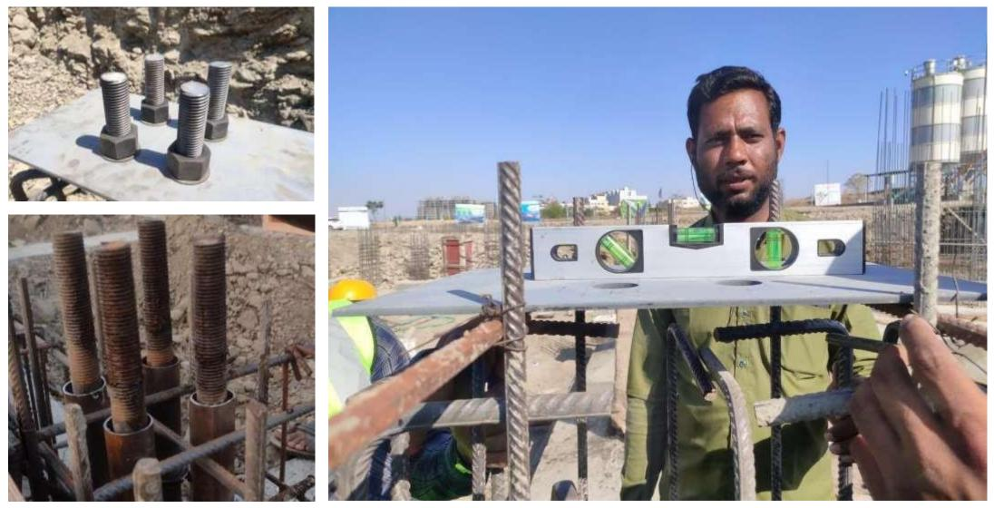
• Fixing of anchor bolts with templates over which factory made built up columns with base plate will be erected.
