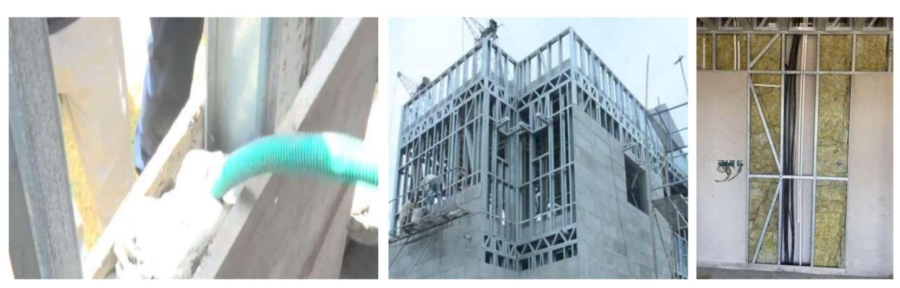
Structural connections of LGSF panels
