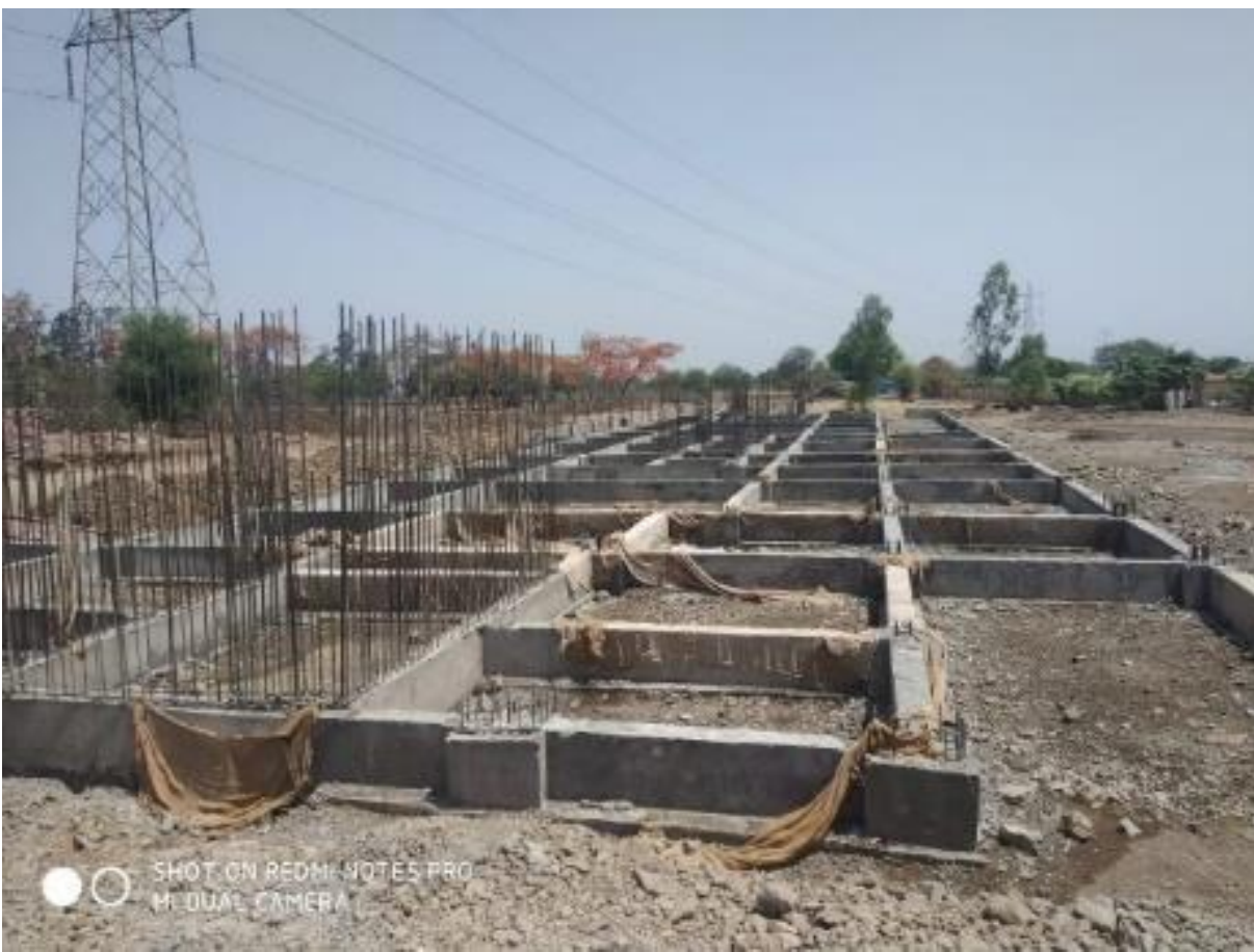
RCC COLUMN UP TO PLINTH LEVEL
