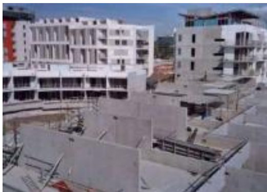
Installation of panels
