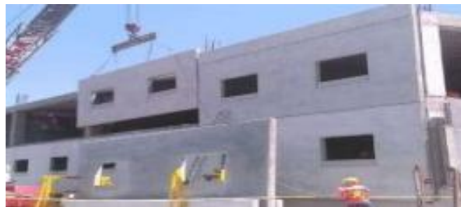
Precast concrete wall (Panels)
