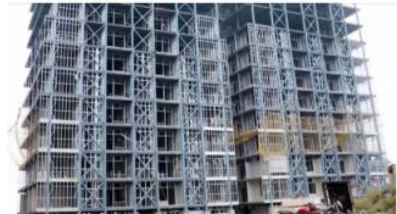
Assembly of LGS Frames and Construction of Wall
