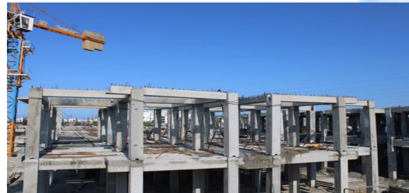
First Floor Column & Beam Erection - May 2021
