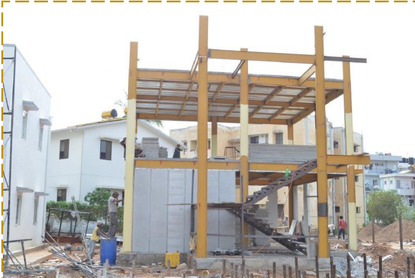
Steel skeleton with Aerocon panel infills
