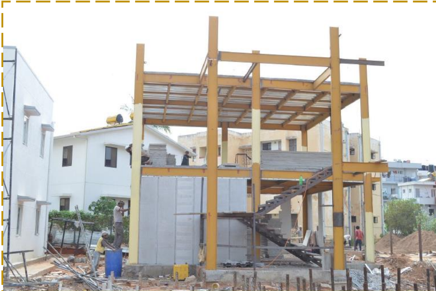
Steel skeleton with Aerocon panel infills
