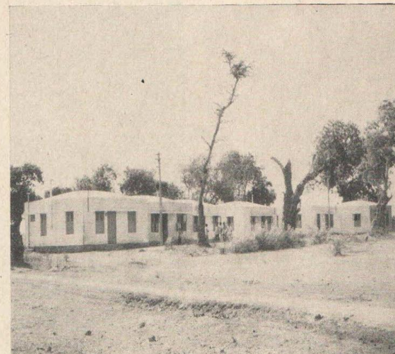
Houses with brick funicular shell roofs at Tada, Andhra Pradesh
