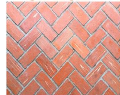
Fig. 2.47. Raking bond.
