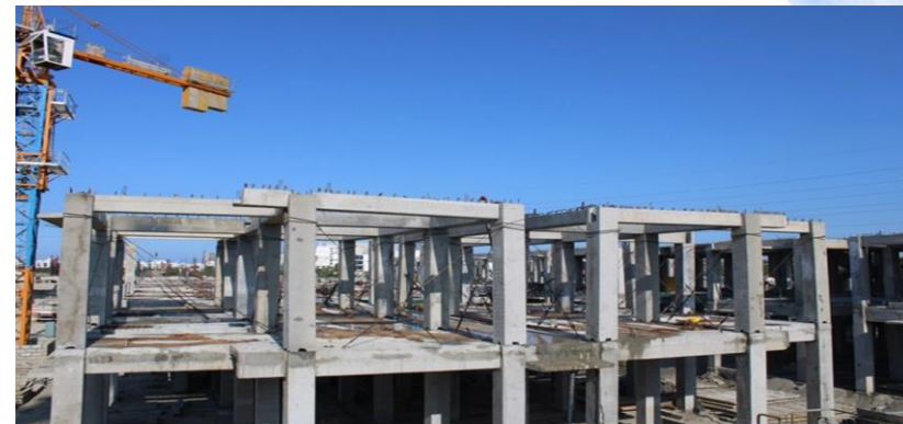
First Floor Column & Beam Erection - May 2021
