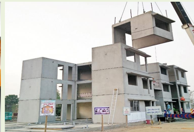
3. 3D Volumetric, Precast concrete construction system (Ranchi, Jharkhand)
