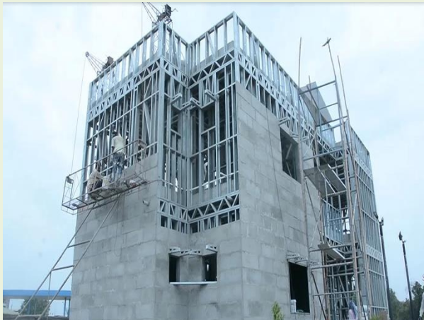
5. Light Gauge Steel Structural System & Pre-engineered Steel Structural System (Agartala, Tripura)
