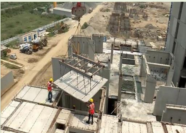
4. On-site assembled Precast concrete construction system (Chennai, Tamil Nādu)
