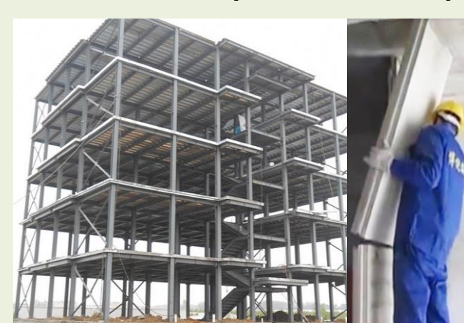
6. Precast fabricated sandwich panel system (Indore, Madhya Pradesh)
