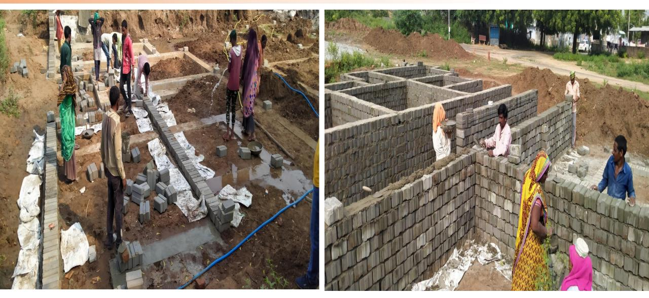
HYDRAFORM BLOCK WALL MASONRY WORK AT FOUNDATION LEVEL WITH MORTAR
