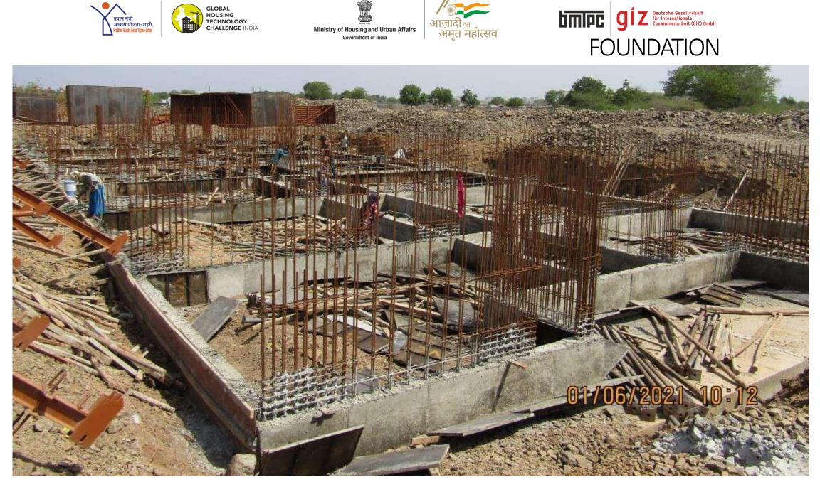
• Plinth beam is constructed above the shear wall.
