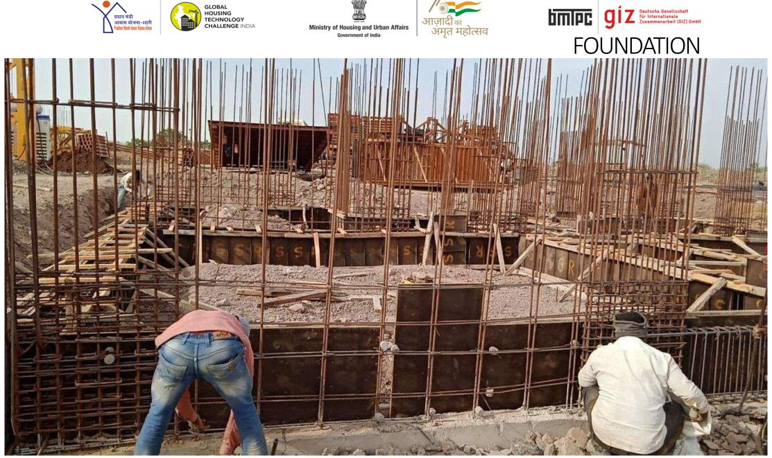
• Plinth beam is constructed above the shear wall.
