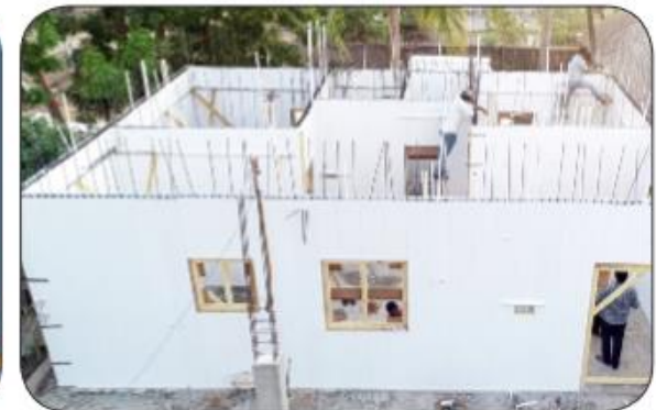
6. Stay In Place Formwork System
