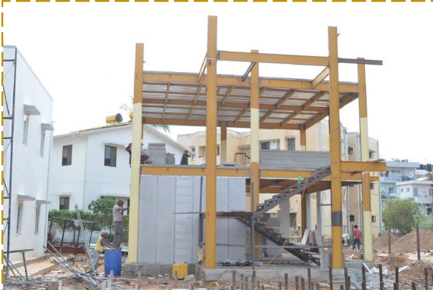
Steel skeleton with Aerocon panel infills
