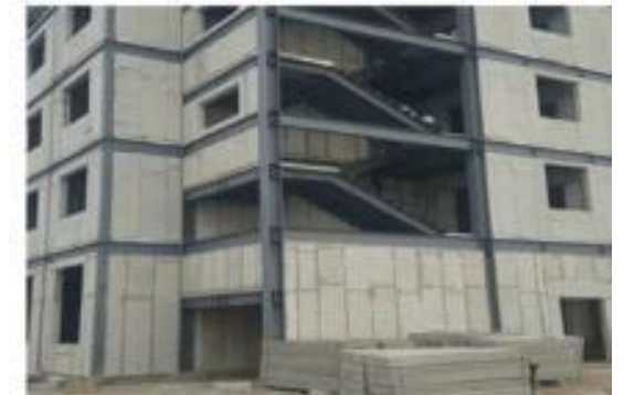
Steel Structure Prefabricated EPS Panel
