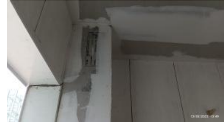
Structure Cover with Cement Fiber Board
