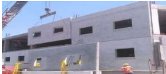
Precast concrete wall (Panels)
