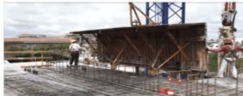
Kicker form of tunnel formwork panel
