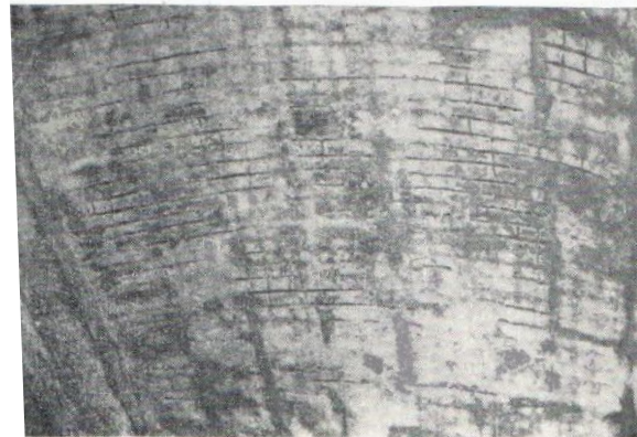
Corrosion damage to an Exposed ceiling of shell Roof
