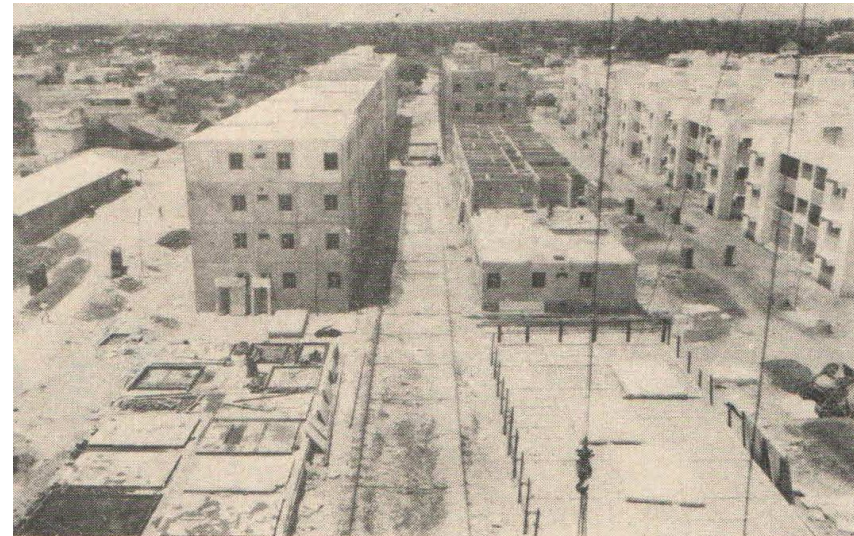
A view of the housing project at Madras using large panel prefabrication developed by SERC
