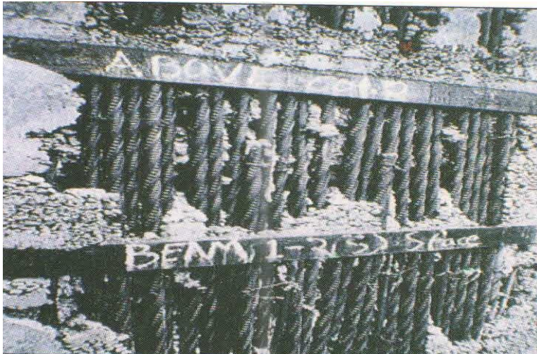
Incorrect planning & placing of reinforcement steel causes segregation concrete
