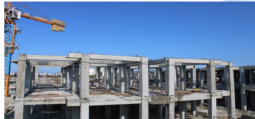
First Floor Column & Beam Erection - May 2021
