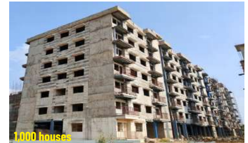
Agartala - nearing completion
