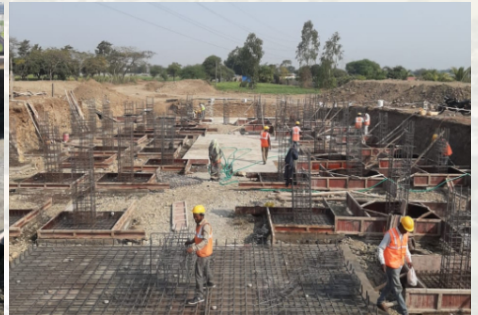
Excavation, laying of PCC, casting of footings and erection of reinforcement for columns in Foundation
