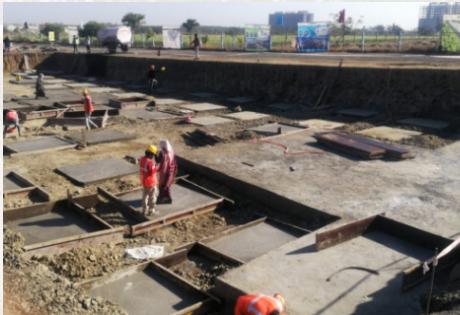
Excavation, laying of PCC, casting of footings and erection of reinforcement for columns in Foundation
