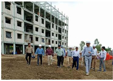
In Indore, 1,024 houses, spread across 8 towers, are being constructed under LHPs. An already established technology named Prefabricated Sandwich Panel System with Pre-Engineered Steel Structural System has been adopted for construction purposes. This technology brings speed in construction, helps in water conservation. It replaces conventional brick and mortar walling construction practices.
