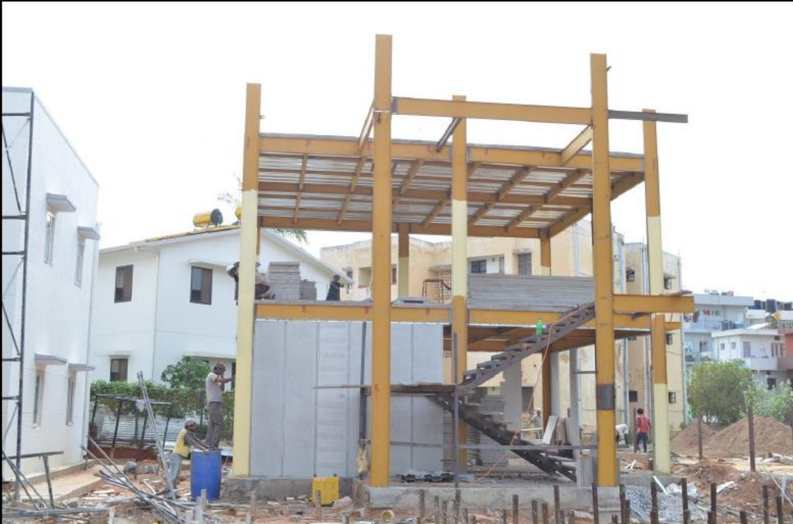
Steel skeleton with Aerocon panel infills
