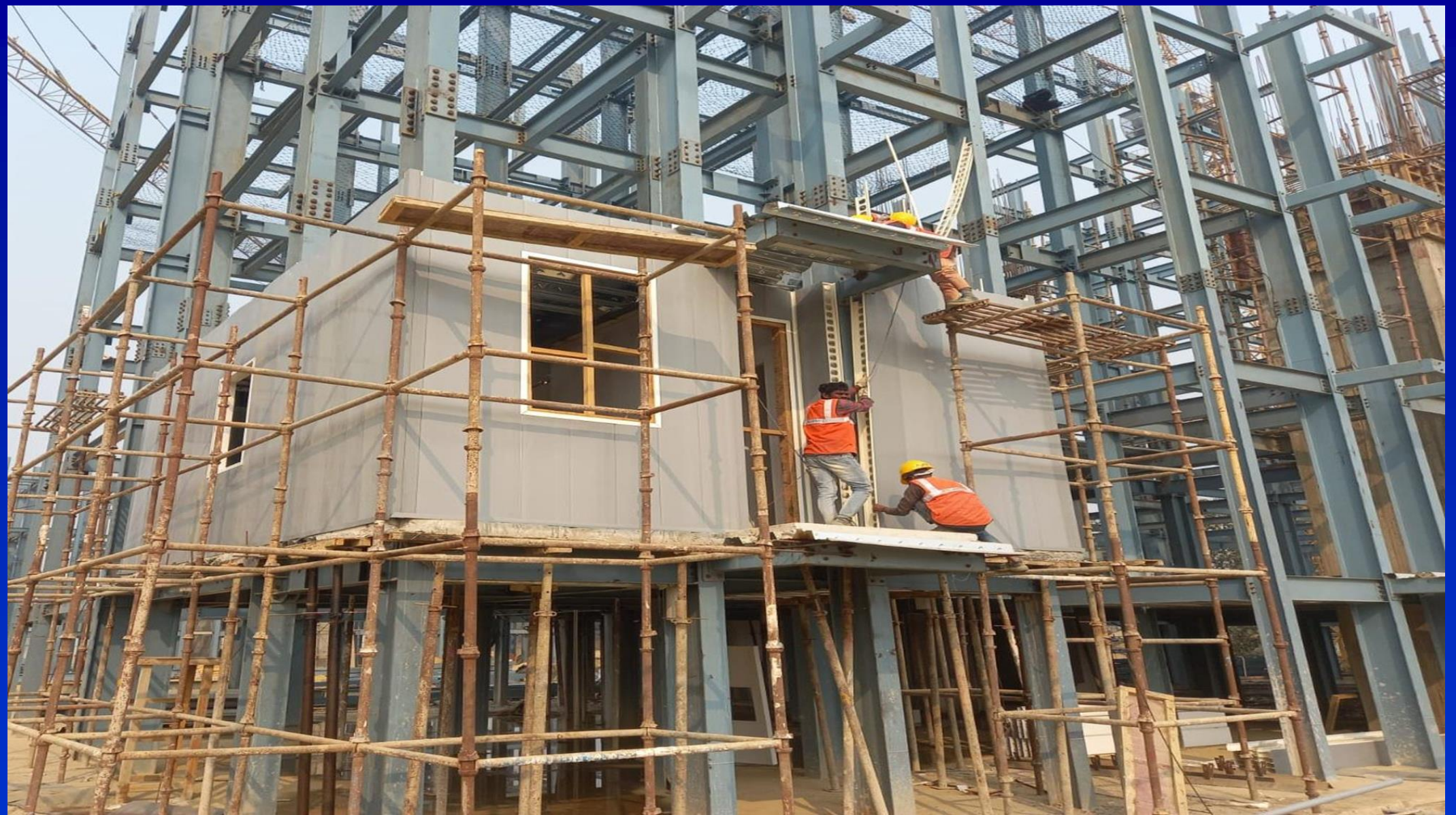
Fixing of Wall Profiles
