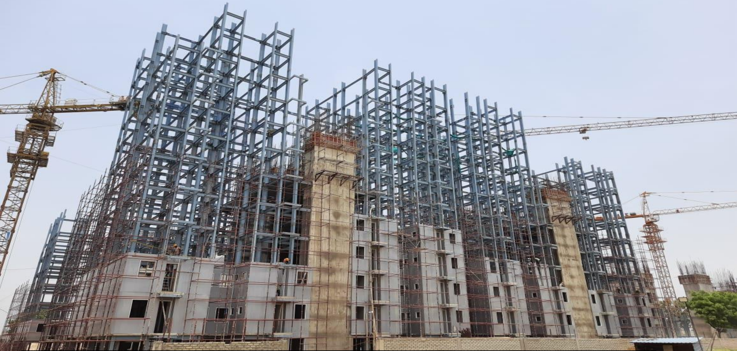
A view of block (A) with shear wall and PEB structure
