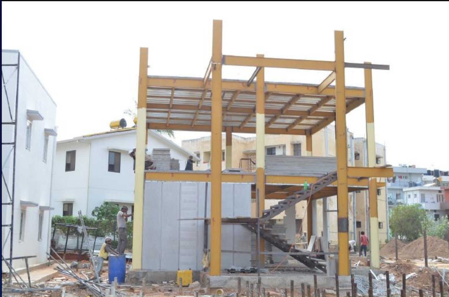
Steel skeleton with Aerocon panel infills
