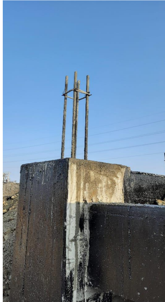
Grouting of beam – column joint
