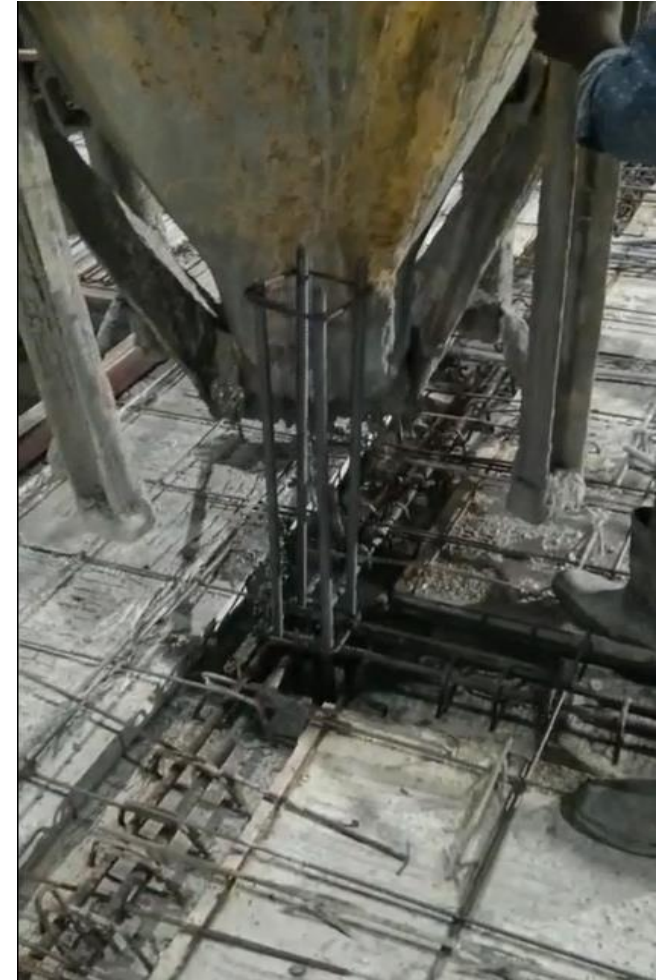
Beam – column - slab wet jointing
