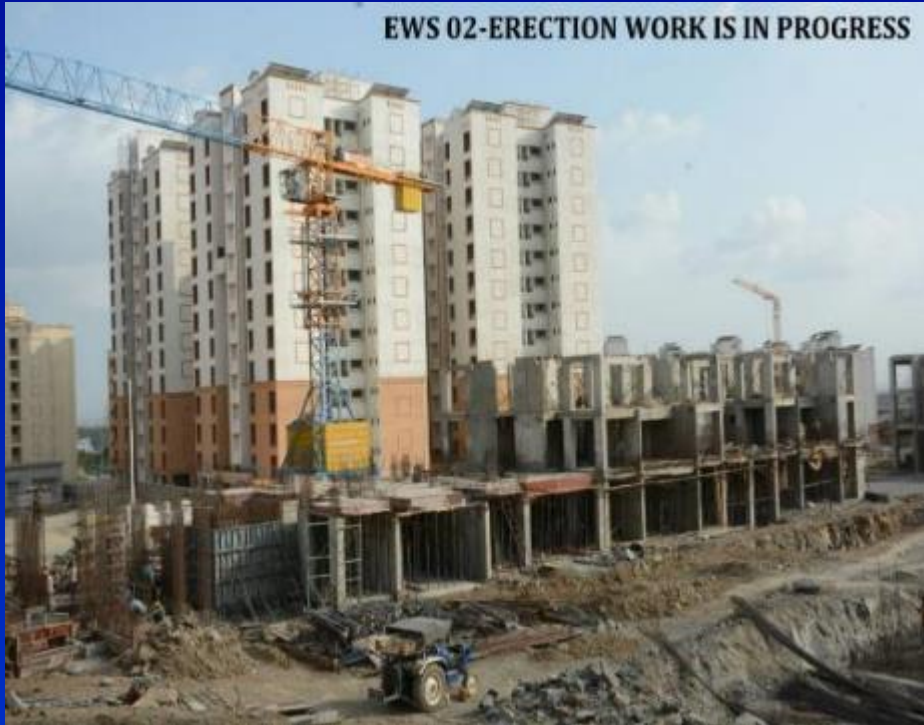
AHP houses in Pune, Maharashtra using Precast Construction Technology
