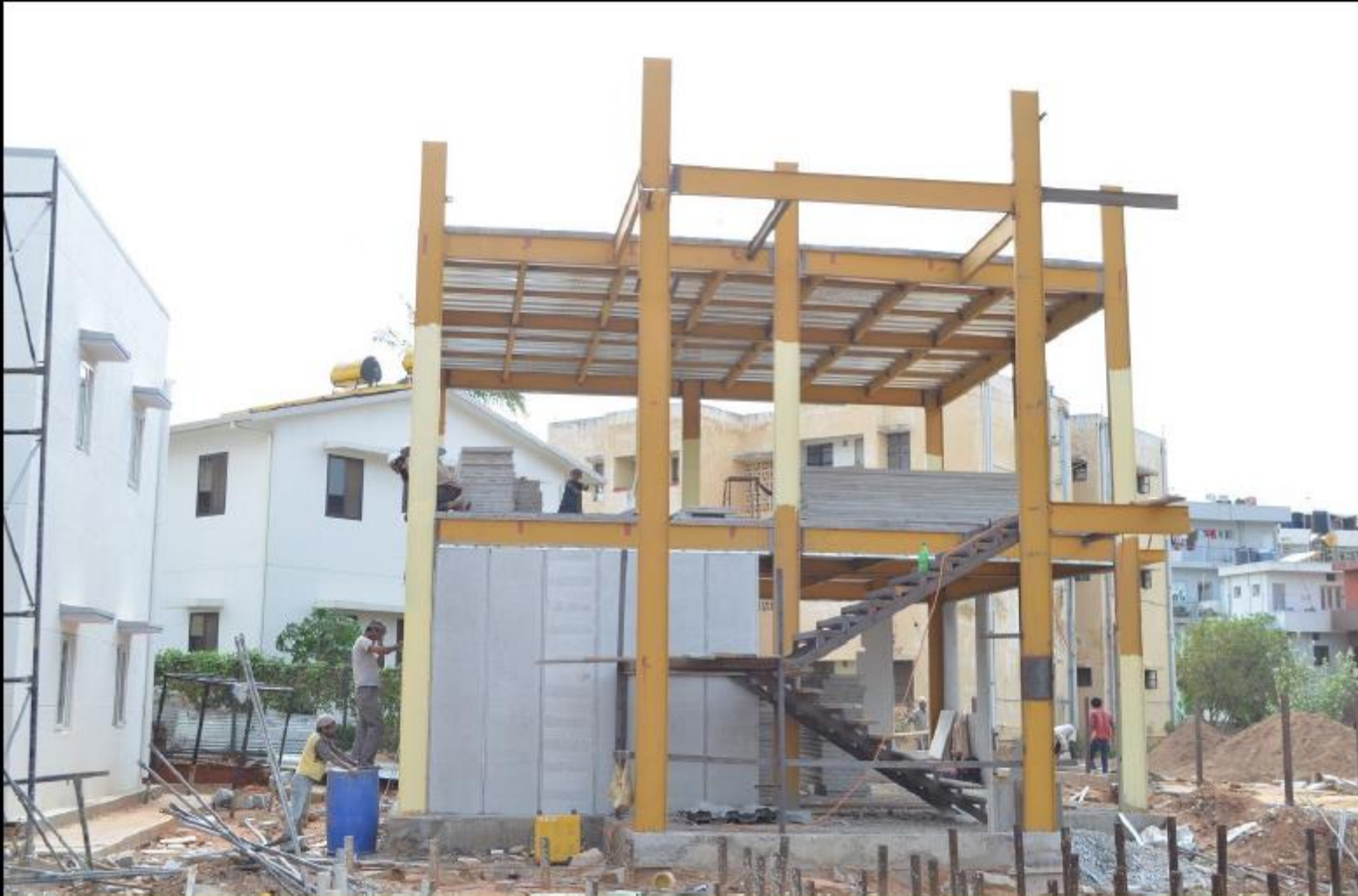
Steel skeleton with Aerocon panel infills
