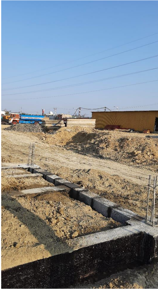
Wet jointing of stem column with plinth beam
