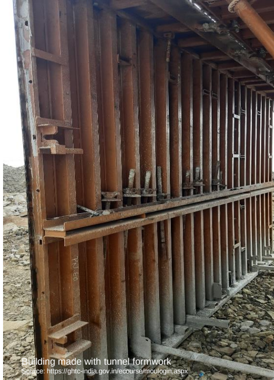
Building made with tunnel formwork Source: https://ghrc-india.gov.in/ecourse/moulogin.aspx
