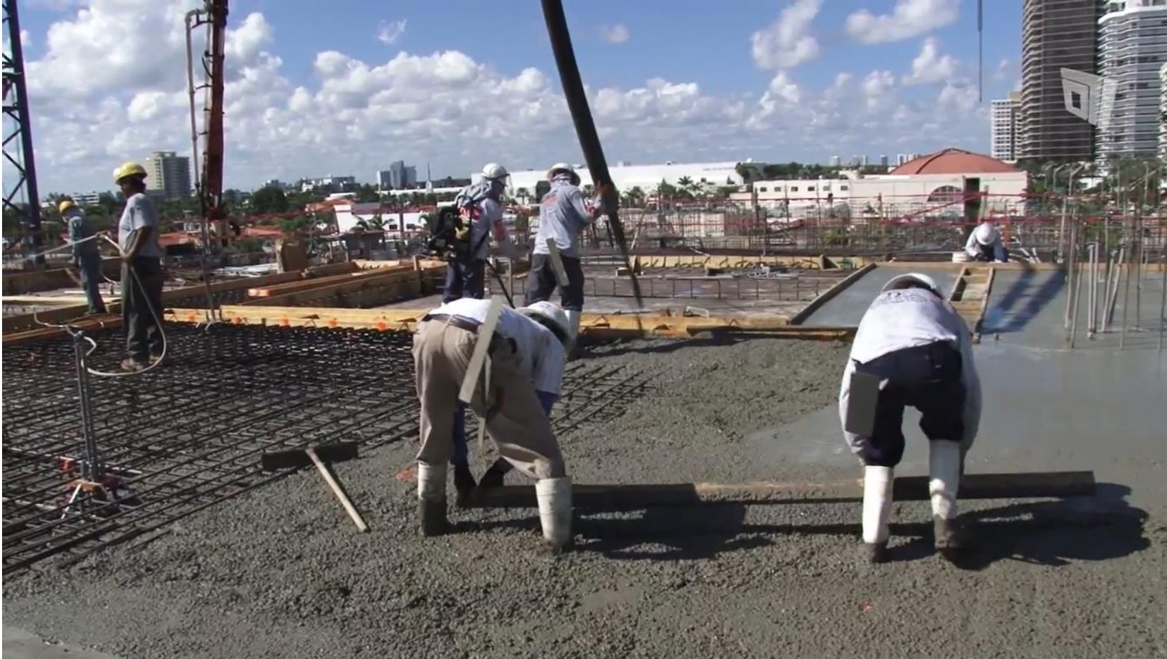
Placement and leveling of concrete
