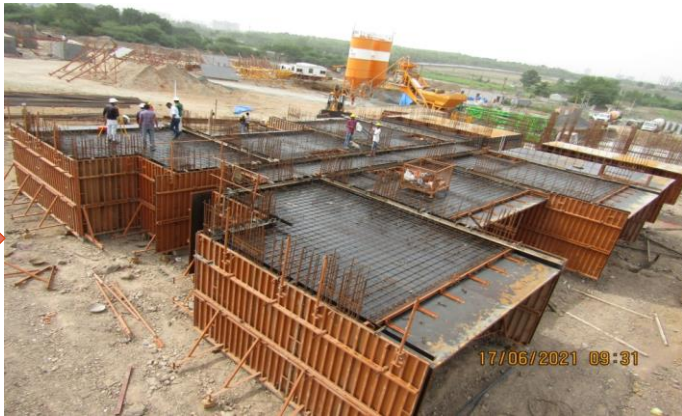
Assembly of Formwork
