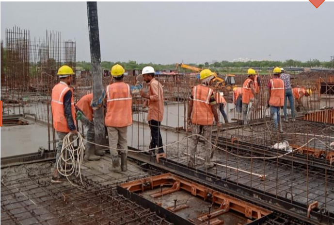
Concreting after Placing formwork
