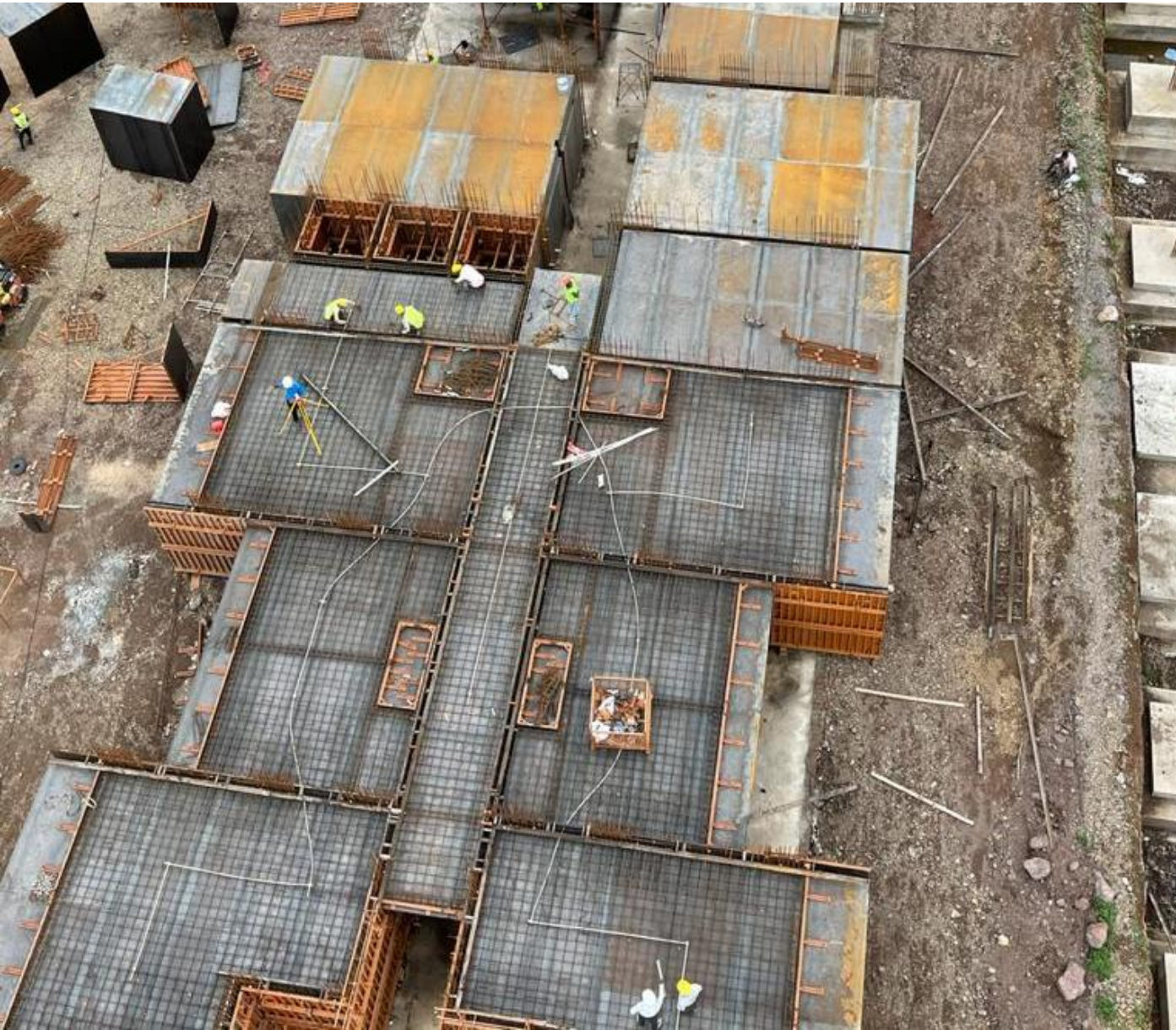
Typical Reinforcement at Slab level
