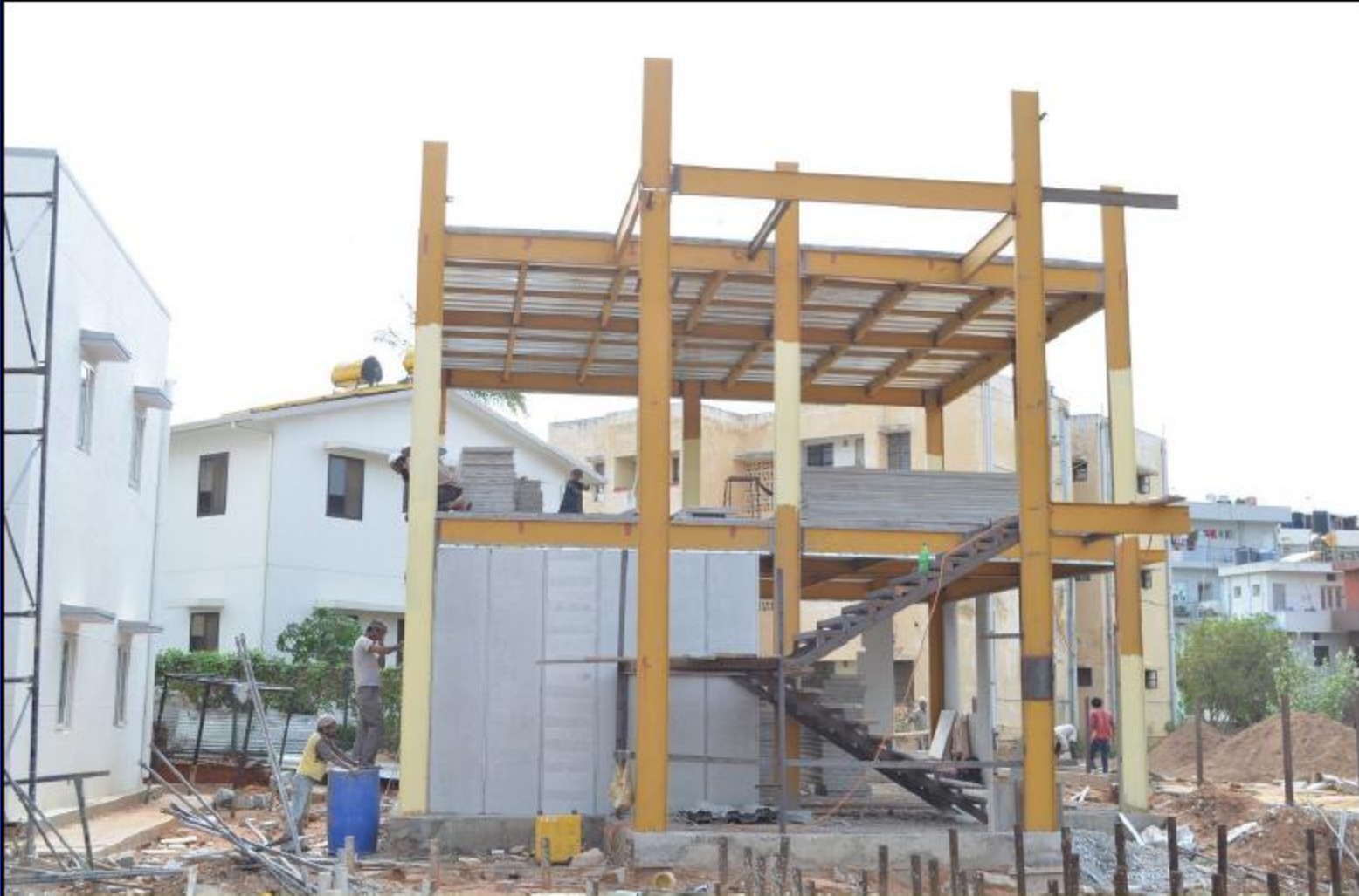
Steel skeleton with Aerocon panel infills
